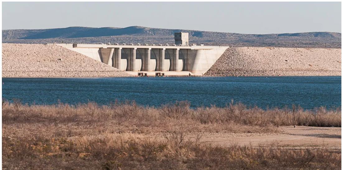
Brantley Lake State Park, with Brantley Dam in the background.
