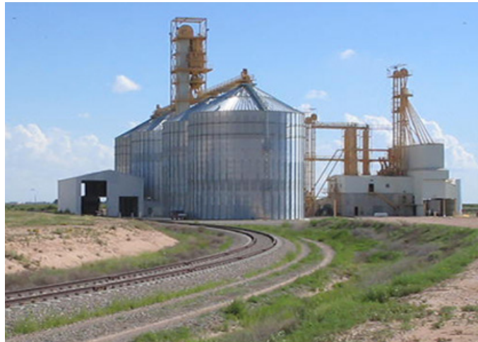
Silo along the rail line.
